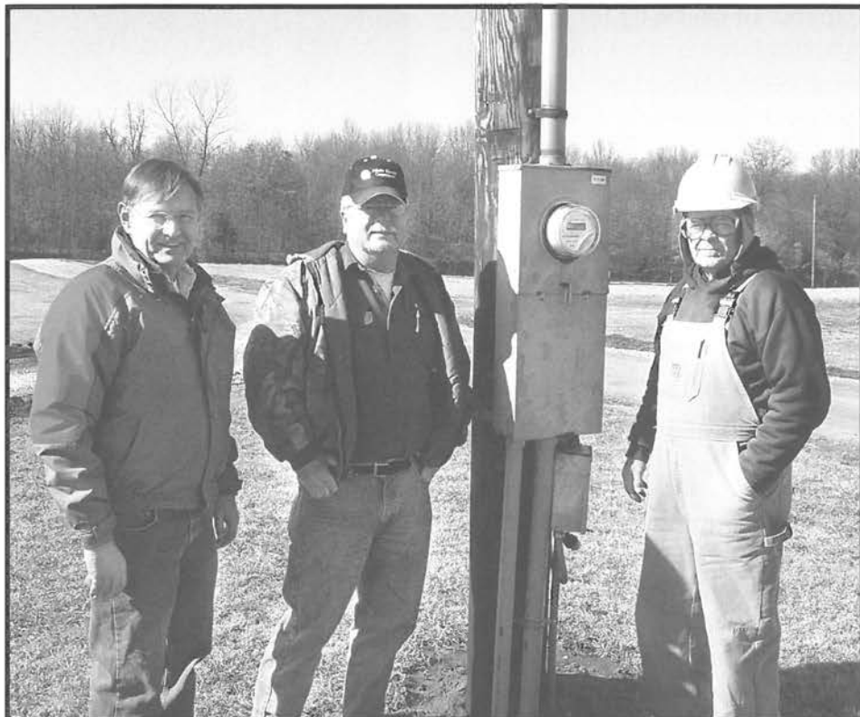
Meter Technician Butch Passley, Part-Time Laborer Donnie Ward and Journeyman Lineman Bill Alexander stand proudly by their last AMR installation. Butch, Donnie, Bill and Buzz (pictured left) dedicated many hours toward the installation process. Members James L. and Betty Stevens at the final location in Augusta were happy to hear they had AMR. Prior to AMR, the couple had to read three meters including their main meter, an electric heat meter and a grain bin at a separate location.
