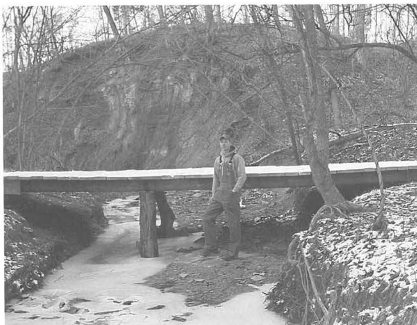
David Croxtan stands next to the finished bridge at Jensen Woods Camp.
