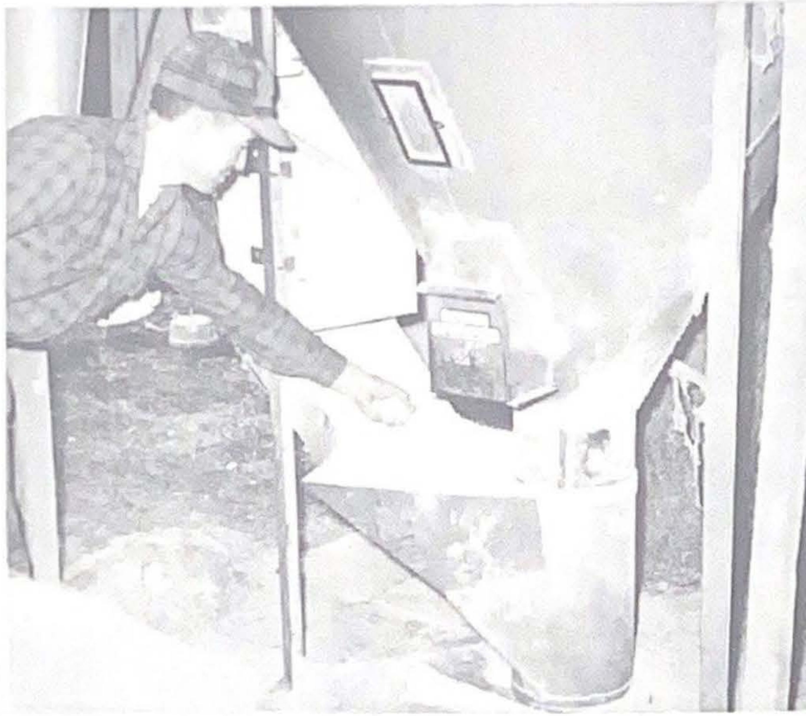
Measuring device dumps ground corn into feed mixer.
