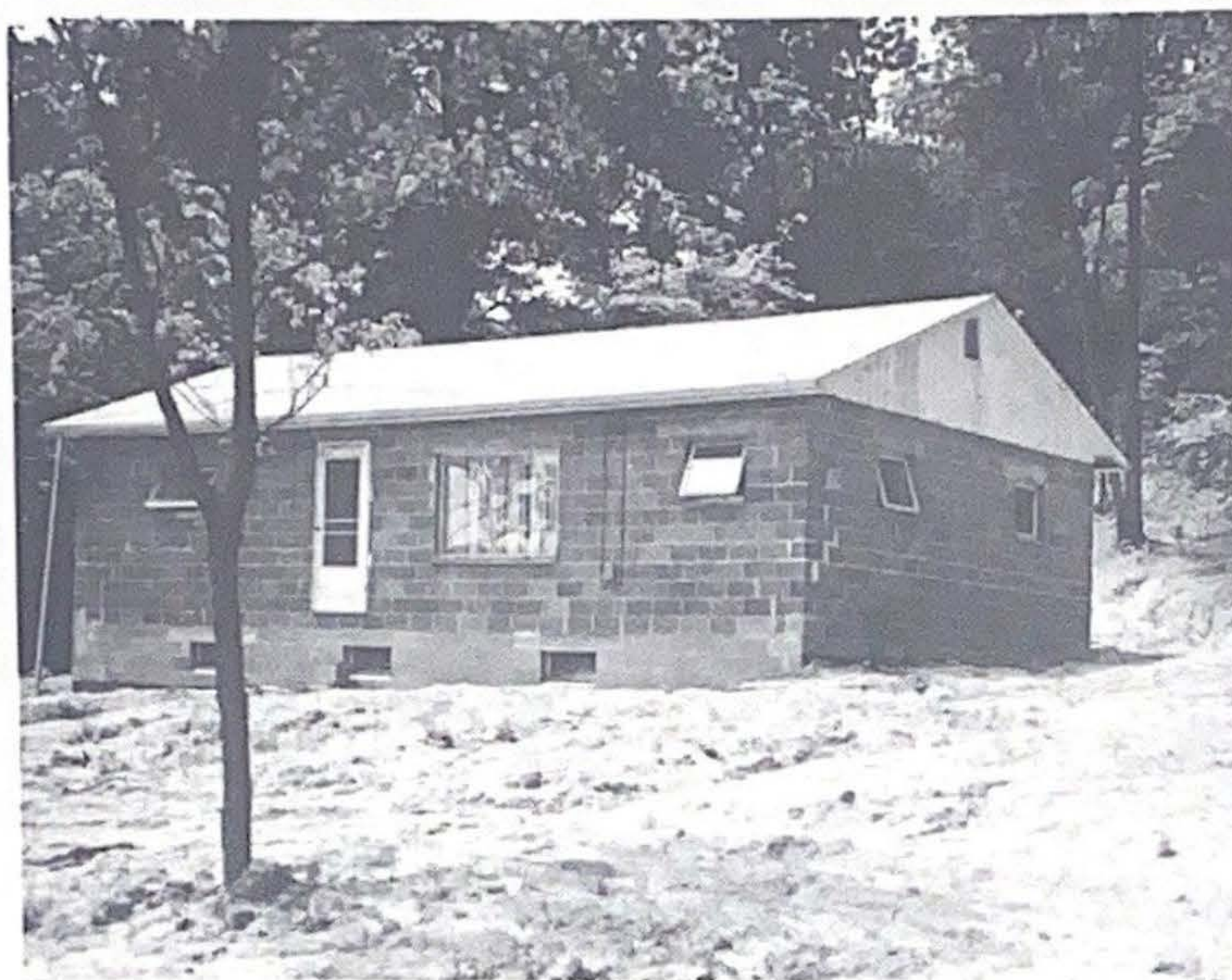
New home of Mr. and Mrs. Robert Genenbacher where electric heat was installed.
