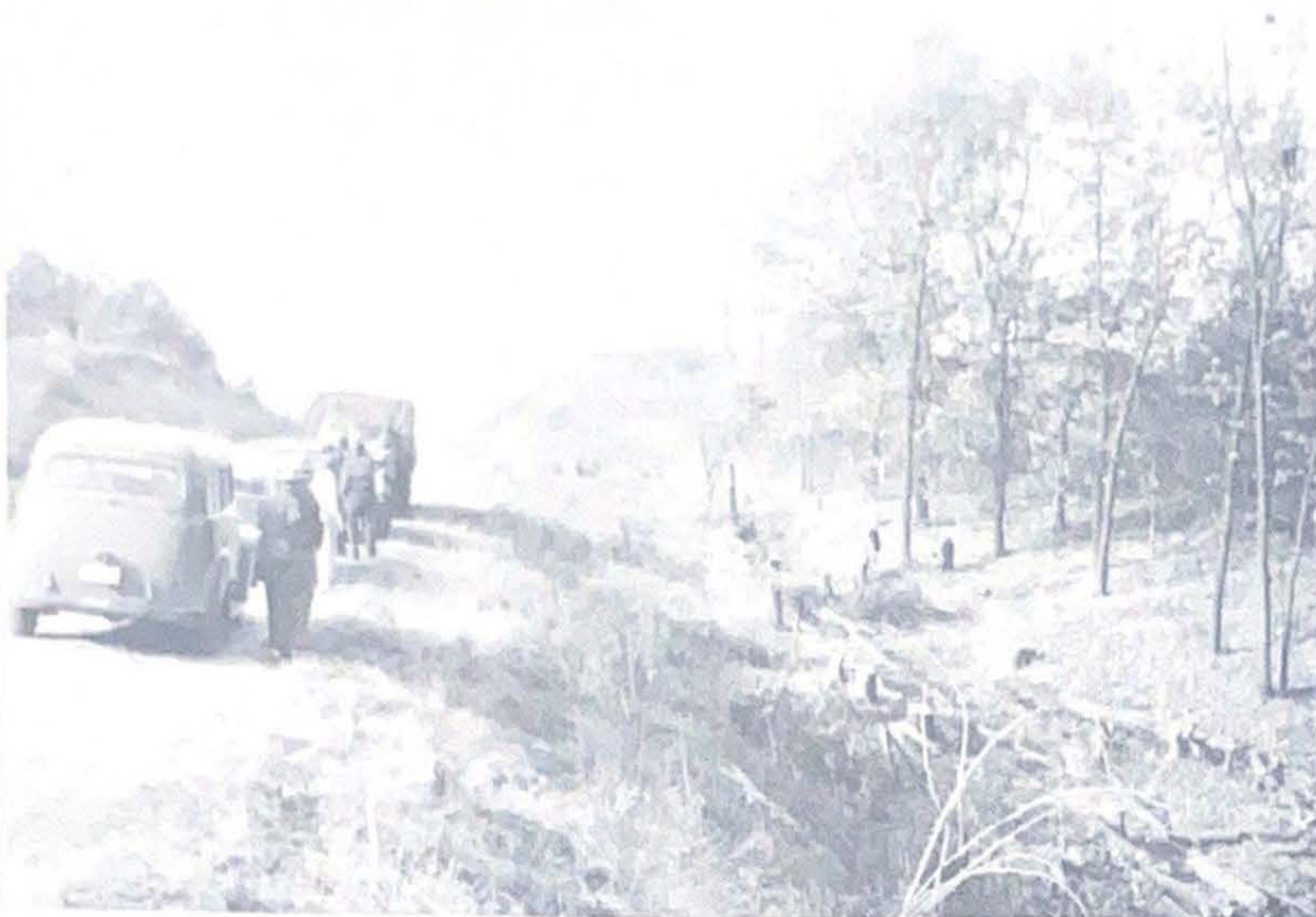
Directors viewing timber being cleared for St. Joseph - Eubanks tie line.
