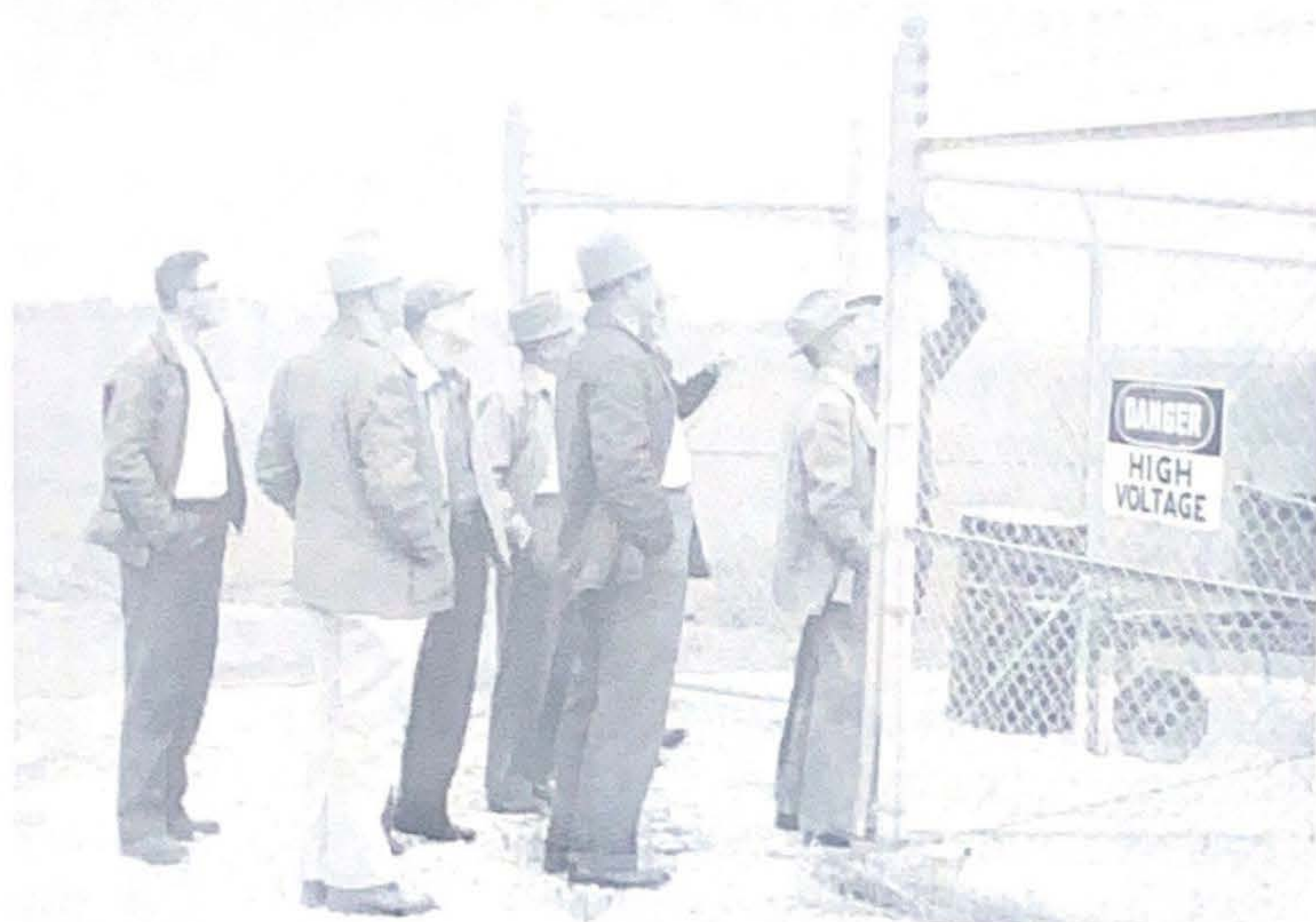
Manager Searls explaining operation of the Ursa Substation.
