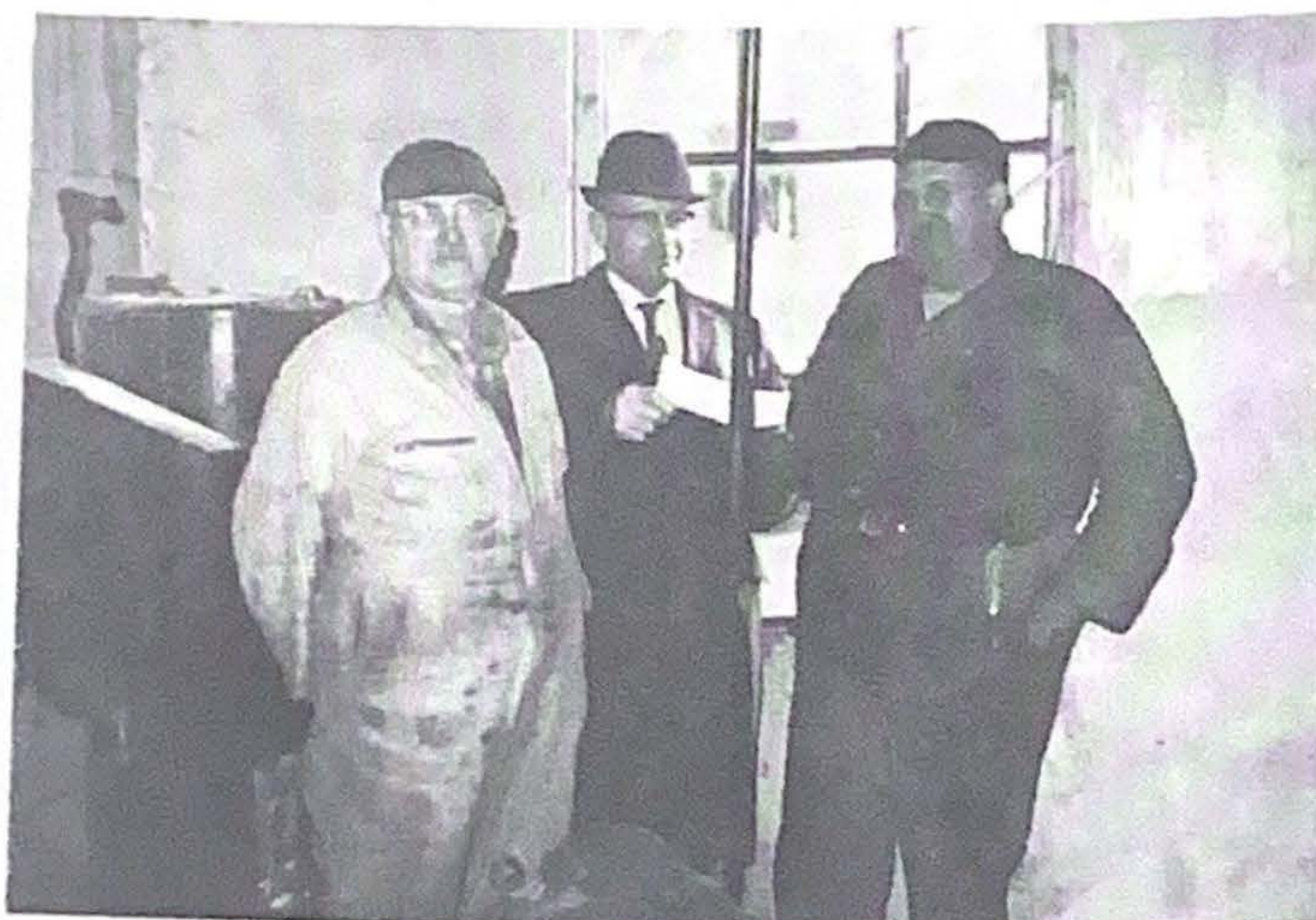
Vice President Harold Bond of Timewell, center, presents check to Mayor Bill Ennen, right, of Clayton. Capital credit check covers service used to operate water filtering, purifying and pumping plant at Clayton Lake. Water Supt. Vern Gallaher is at left.
