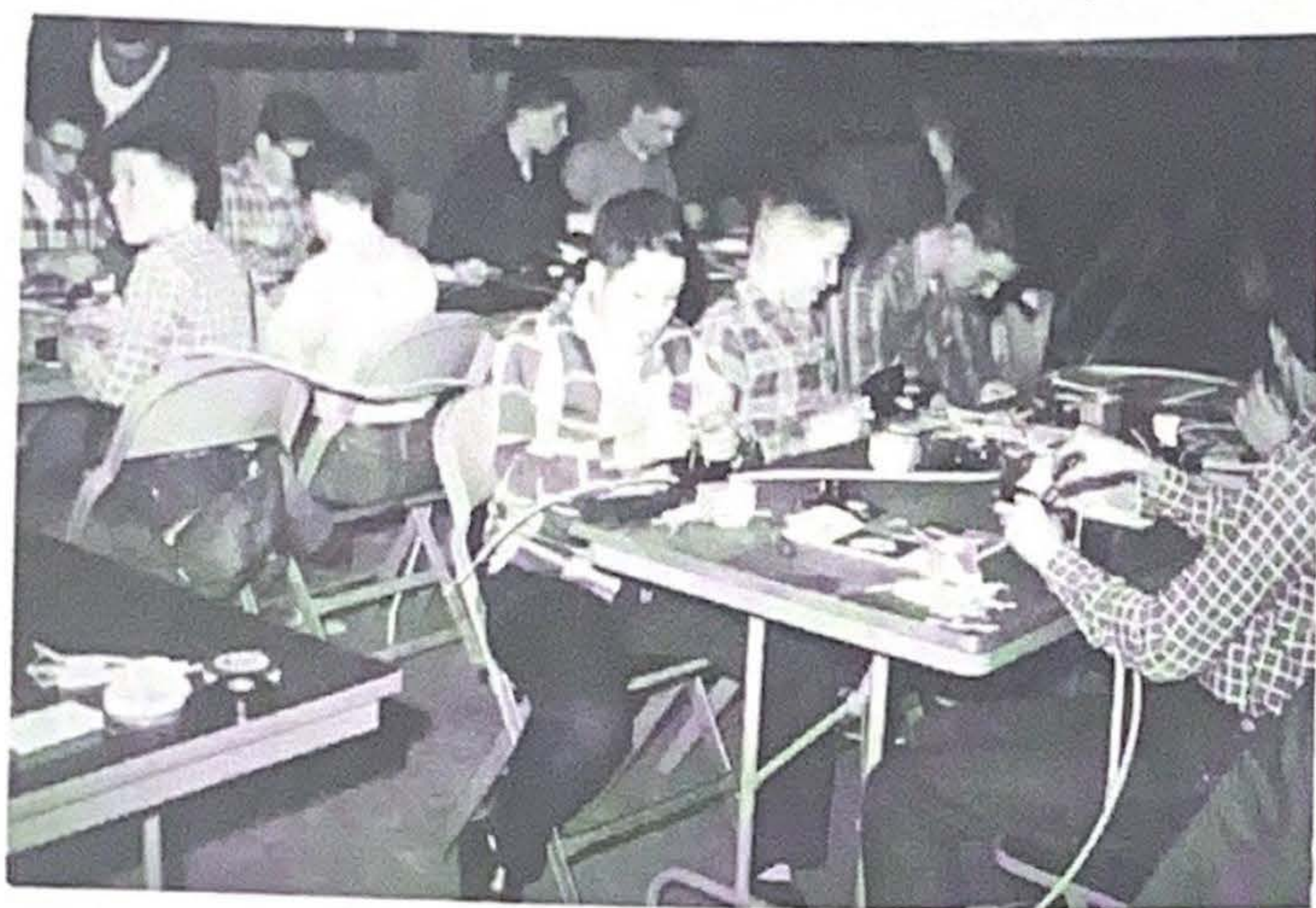
Second year group wiring single pole switches.
