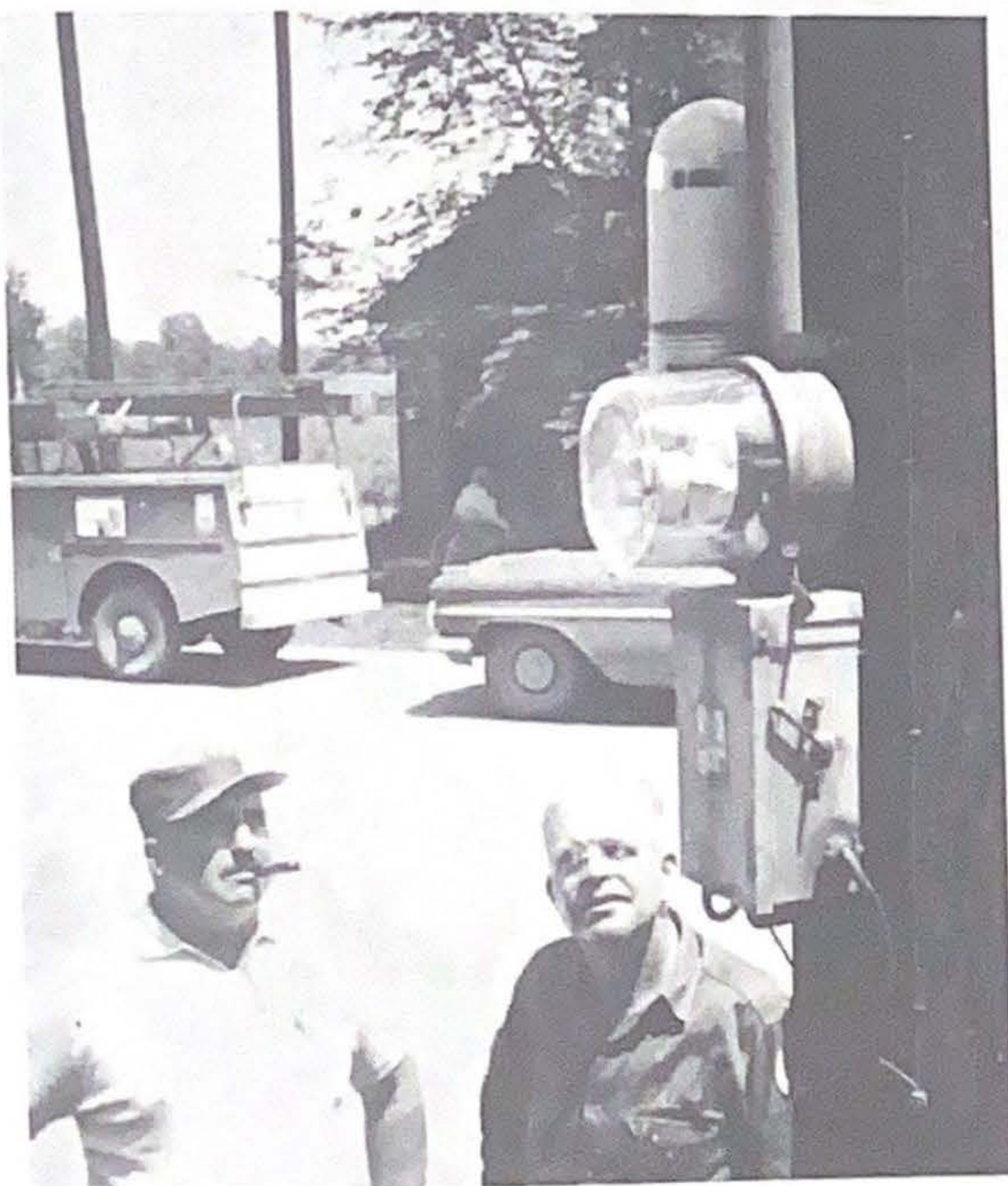
Bill Wear and Co-op employee Alfred Hetrick, discuss automatic control for streetlights. Large glass object behind meter is electric eye which operates lamps according to the light intensity.
