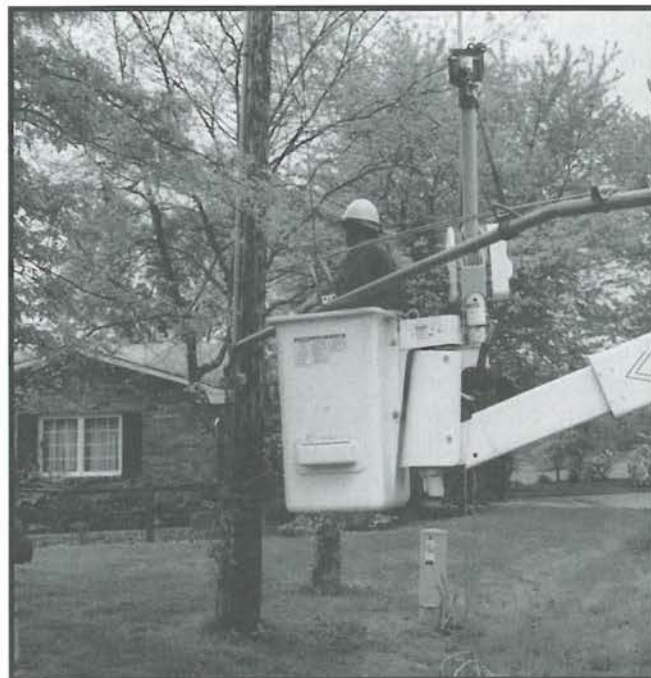
Lineman Charlie Rossiter installs a new 250-watt security light at the intersection of State Street and East Lake Estates Subdivision.
