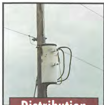
Distribution Transformer
