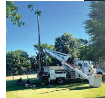
Adams Electric employees Brennan Caspermeyer, Duane Jones, Logan Schutte, Cole Wellman, and Dustin Waddell used their community service hours to install lights at Bailey Park in Camp Point.
