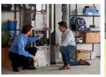
HVAC System Maintenance
