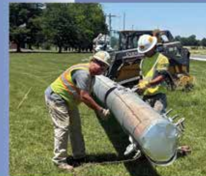
Above: A contractor for PPI prepares a transmission pole for installation.
